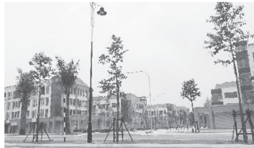
Marina Square Commercial Centre, Miri
