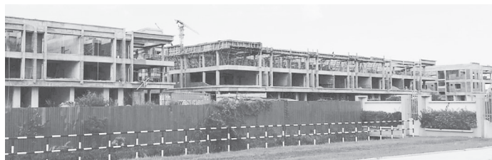
TT3 Commercial Centre at Jalan Canna, Kuching
