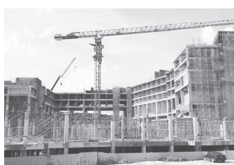
TH Hotel along Jalan Lapangan Terbang, due for completion by 2016/2017
