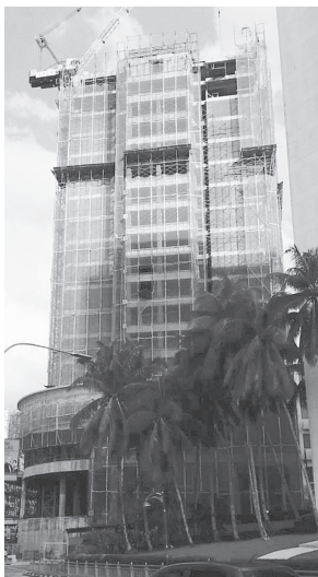
Majestic Tower Hotel (next to the Riverside Majestic) under construction
