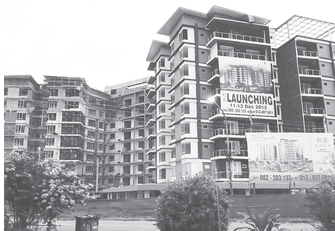
The Royale, 9-storey apartments nearing completion at Jalan Stampin Timur, Kuching
