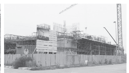
Hotel UCSI under construction at the Isthmus, Kuching
