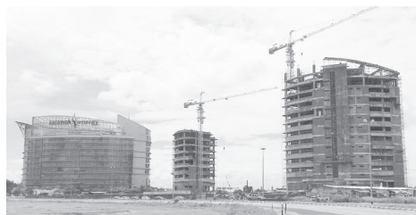
The Gateway Towers, purpose-built offices housing SEDC and LCDA Headquarters at the Kuching Ishtmus
